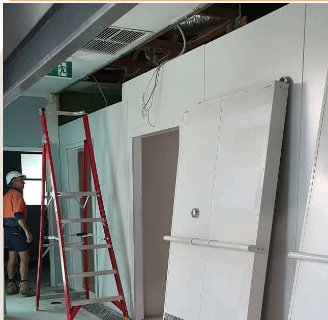
New fridge and freezer in the kitchen
