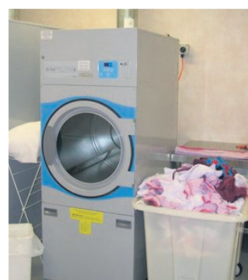
Above: Solar panels assist with water heating. Below: Hot air from clothes driers is transferred to cooler areas in the facility.
